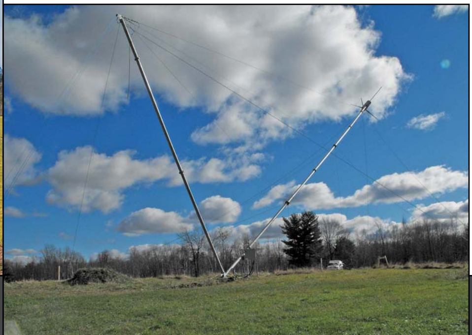
Tilt-up towers require a large, open site to raise and lower the tower, but guyed towers can be sited on cluttered sites and even between buildings.
