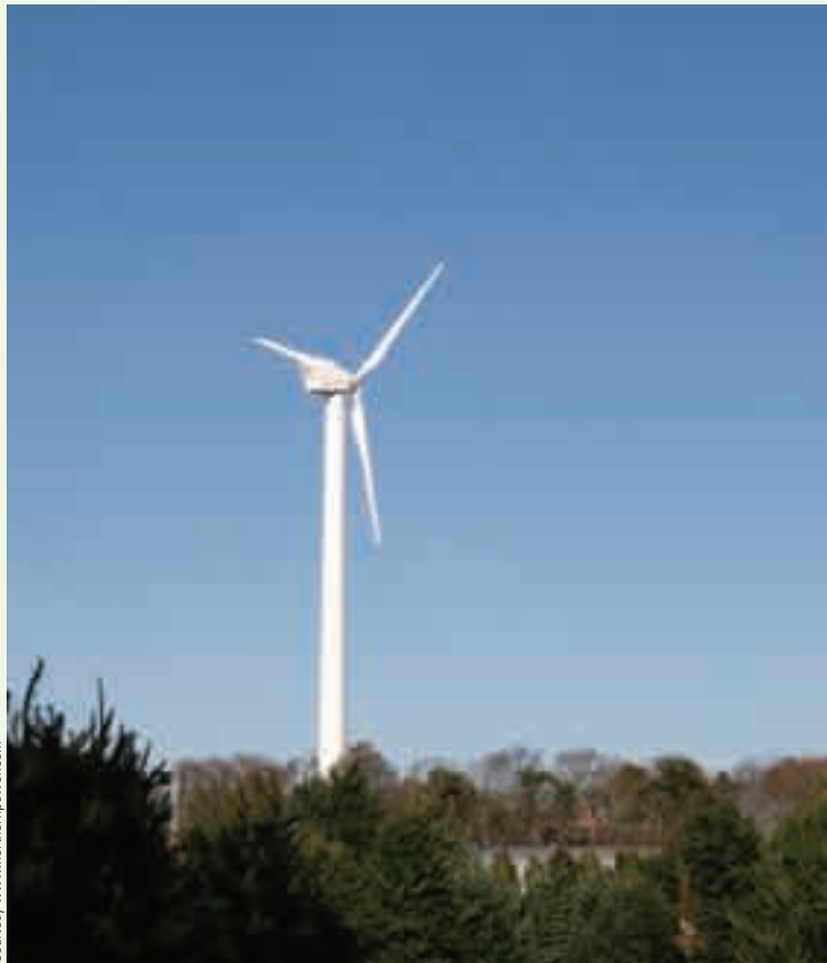
The Northern Power Northwind 100 turbine is the largest turbine included in this guide, with a 69-foot-diameter rotor.
