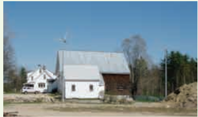
These two wind turbines on very short towers underperform because they are below the area's tree line and very close to obstructions.
