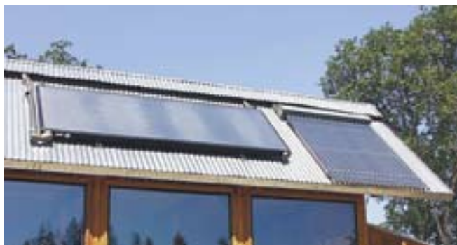
A flat-plate solar domestic hot water collector (left) and an evacuated tube collector (right).
