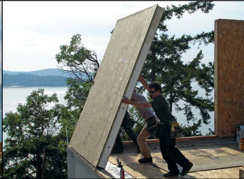
Made of expanded polystyrene and oriented strand board, SIPs are relatively easy to maneuver by hand.
