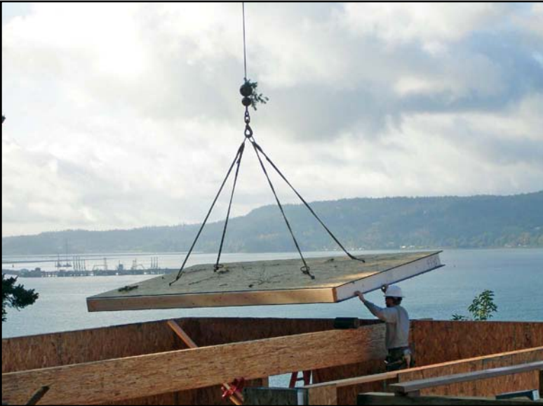
Structural insulated panels for the exterior walls and roof are not only efficient; they also come pre-cut so the house goes together quickly.
