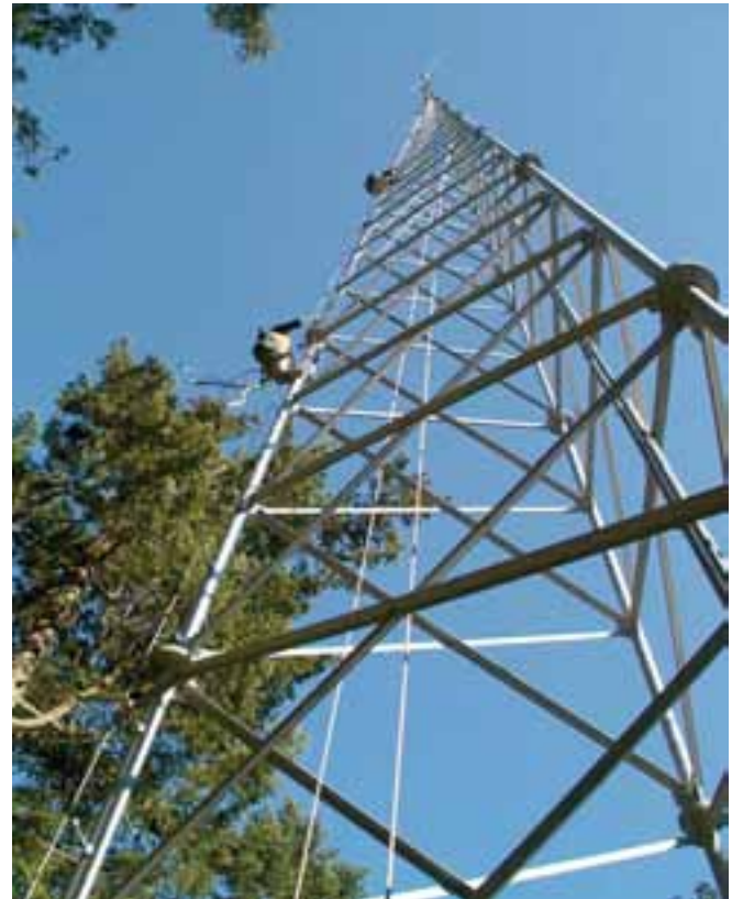
With the wind generator installation complete, it's time to begin installing the PVs.
