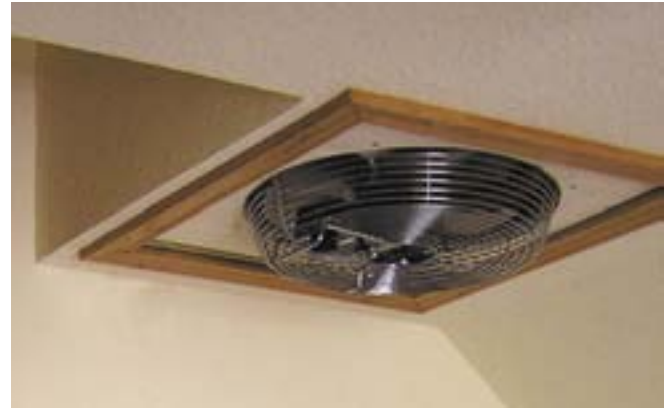
Using a removable whole-house fan eliminated one month of air conditioning use in this Texas home.
